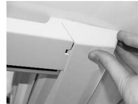
Refit the inner frame covers by locating the securing lugs and keeping the covers parallel against the roof whilst sliding them carefully onto the frame, 'clicking' back into position, without distorting.
