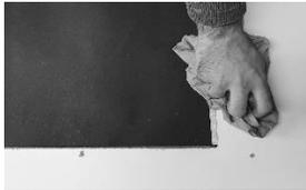
Please clean the frames carefully before mounting the sealant. Remove dirt, grease, oil or release agents from the assembly area.
