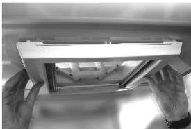
Correctly position the plissé frame to the inner mounting frame and clip it into place. Special centring devices will help to find the right position.
