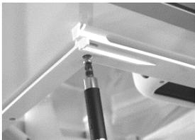
Correctly align the upper frame and the installation frame and secure evenly with the screws.
